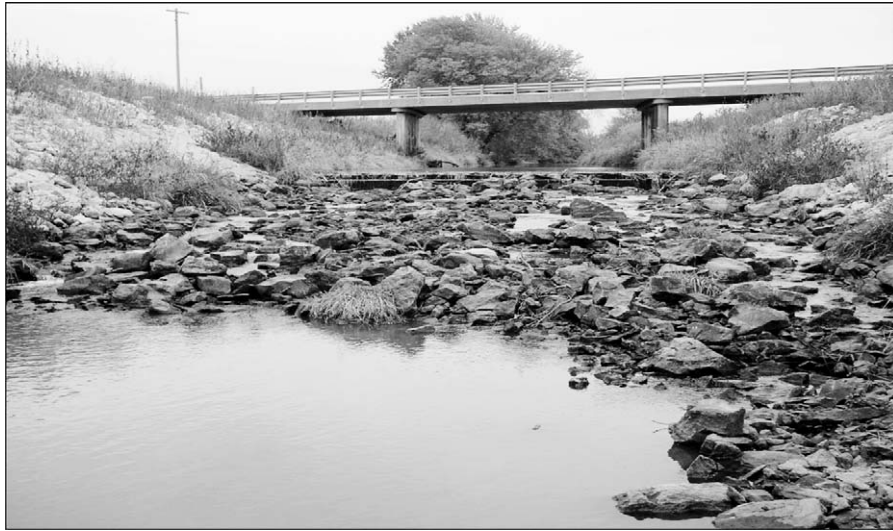
FIGURE 1.—A grade control structure on Turkey Creek at low-flow conditions.
